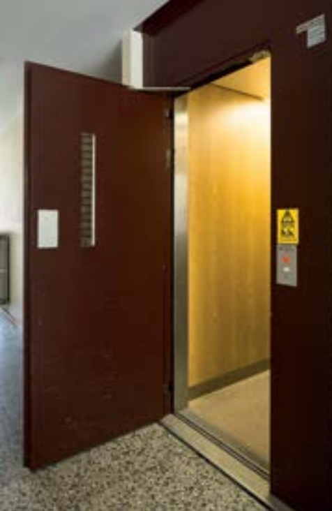
Old elevator before modernization.
